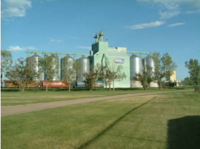
Grain Elevator at Beiseker
